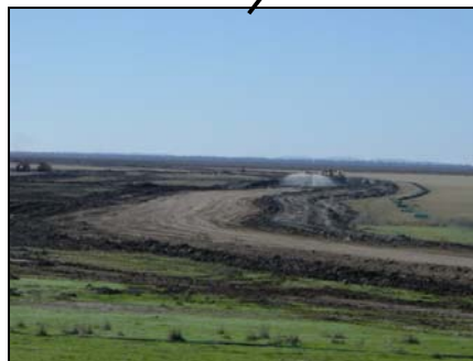
Plate 5: Commencement of Temporary Isolation Bund.
