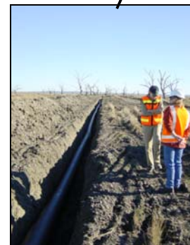
Plate 6: Pipeline trench across Lake Cowal.
