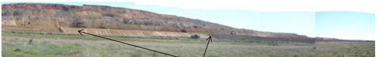
Rehabilitation works adjacent to Pond D1 using the rock-topsoil method for revegetation of the lower batters.
