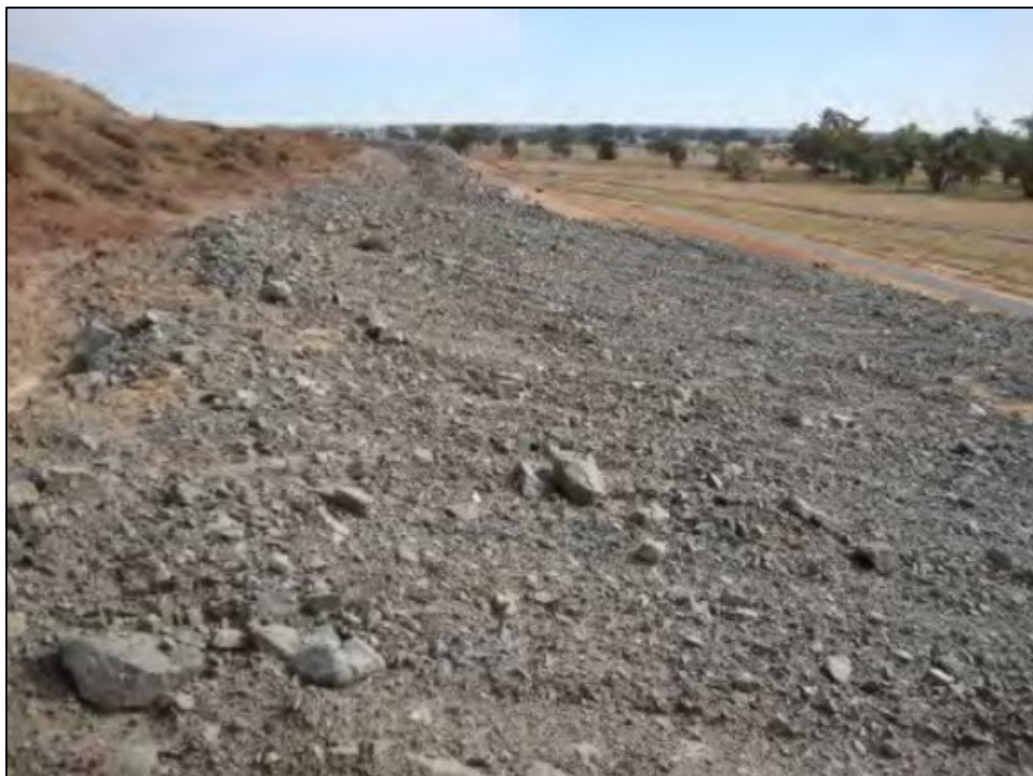
Photograph 1: Topsoil (brown material top left) has been placed above the (grey) rock mulch underlay in preparation for spreading (Photo courtesy of Donna Johnston, DnA Environmental).
