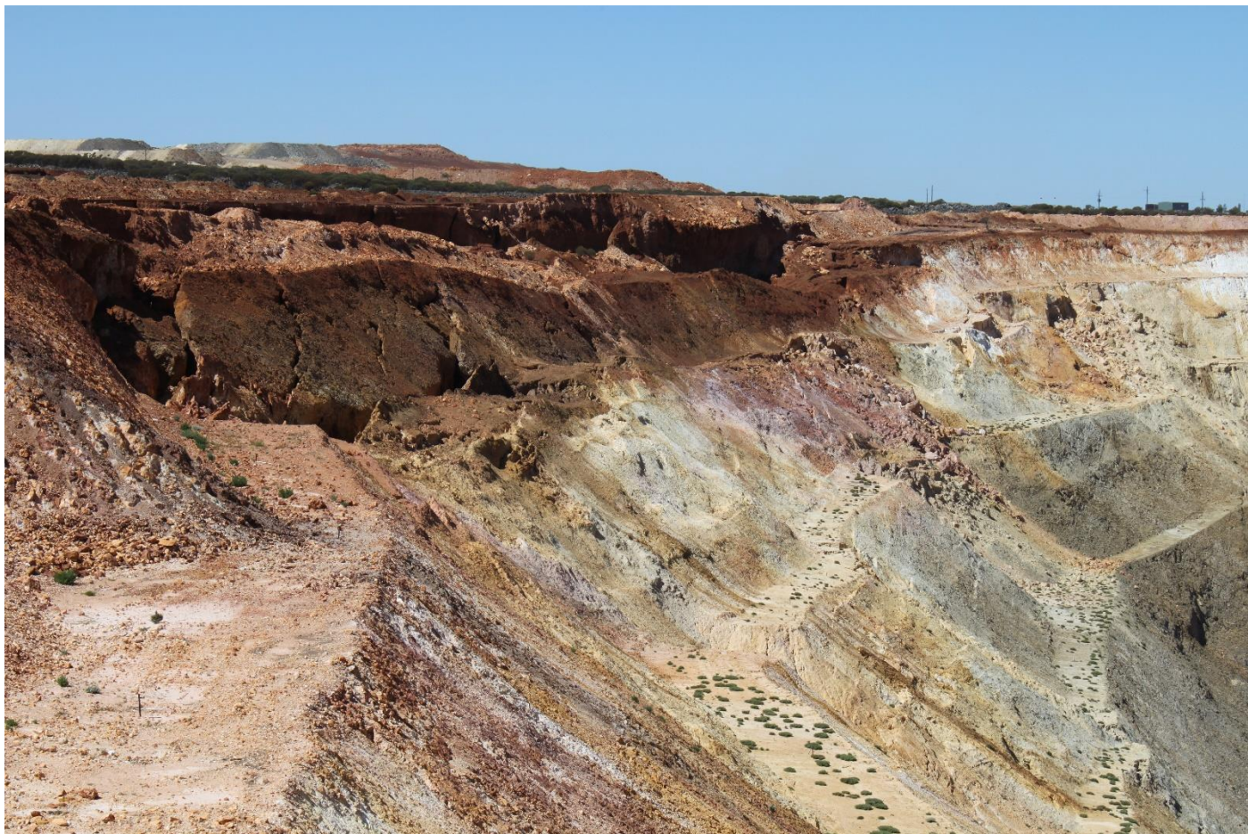
Figure 2-15 Example of surface subsidence following a large-scale slope failure at another mine.
