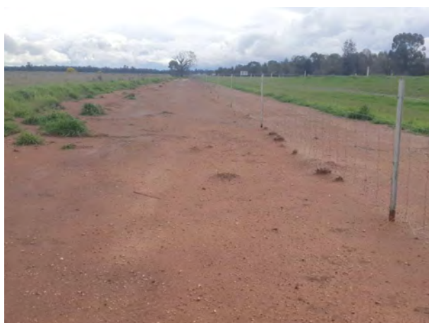
Plate 6.11 Example of sheet erosion on the vehicle access tracks (CGO AS1), view facing west
