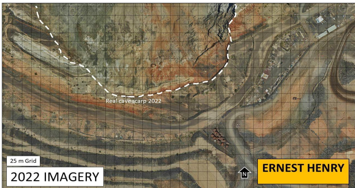
Figure 5-4 Aerial imagery from 2022 showing the zone of subsidence at year 2022 (i.e., existing conditions at 2022)(Beck Engineering, 2023a).
