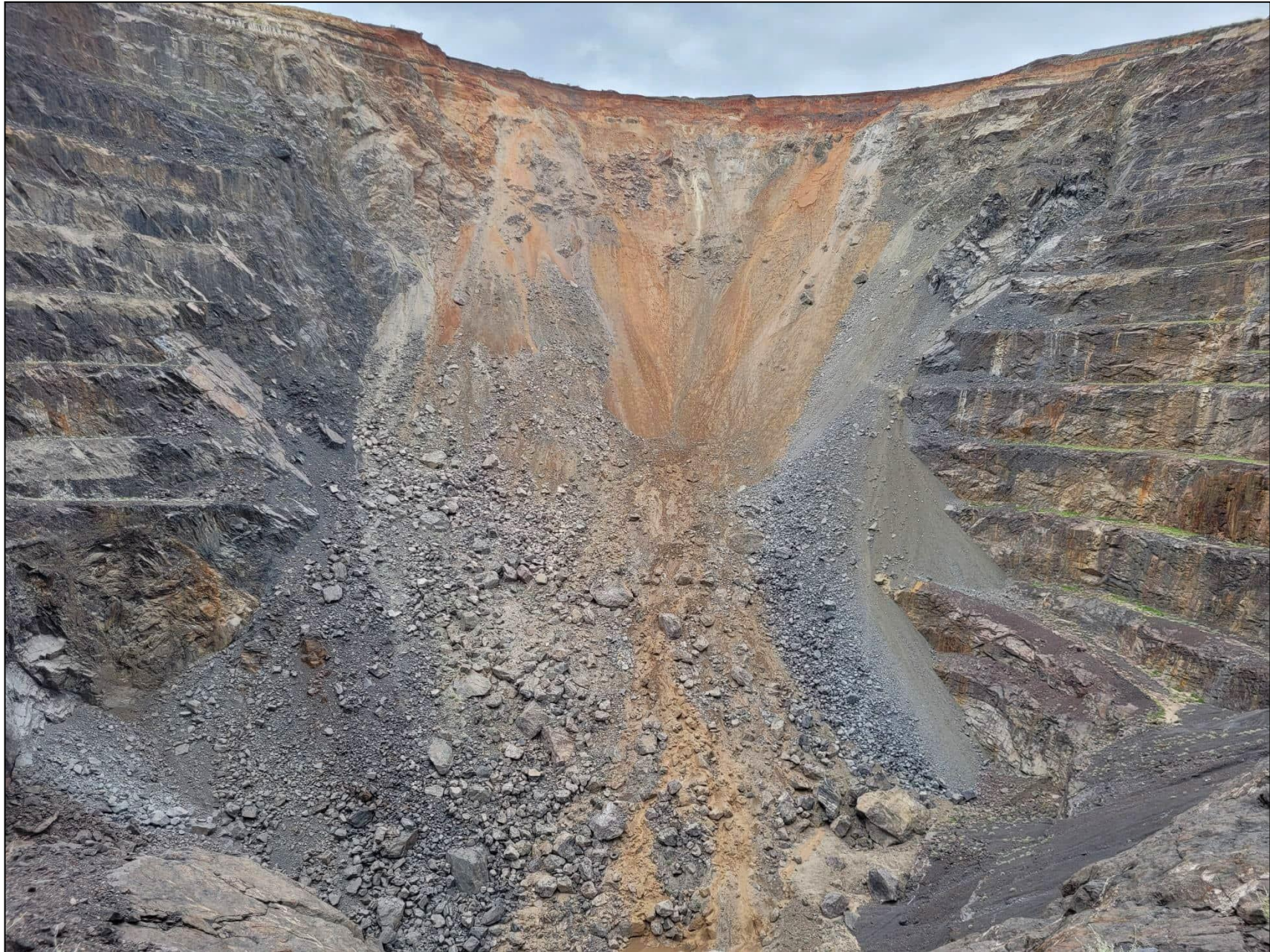
Figure 3-3 South wall of the Ernest Henry open pit and cave zone (photo taken January 2023).
