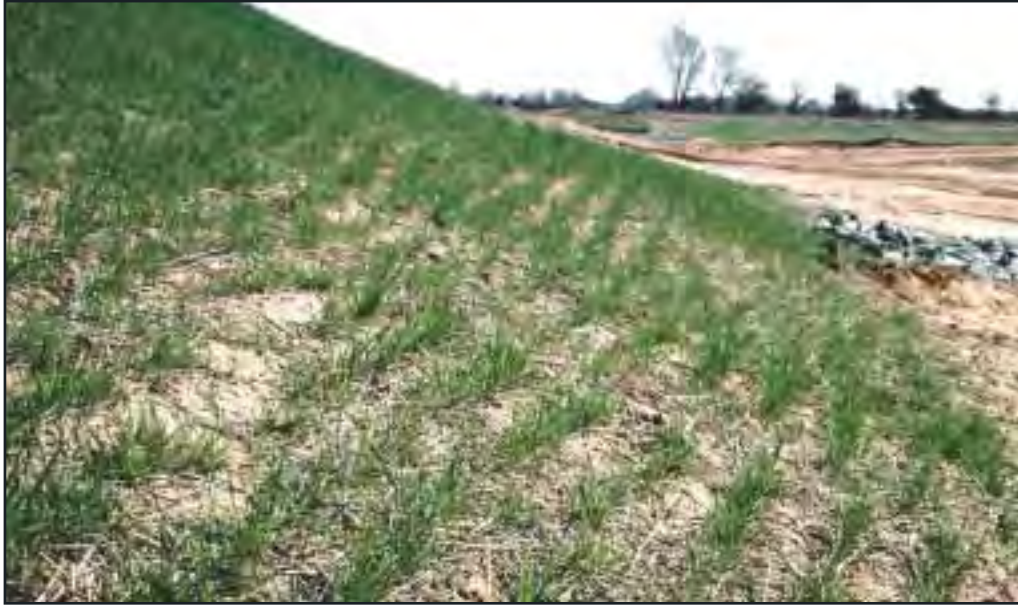
Figure 4.3(b) A track-walked slope (see footnote 4)
