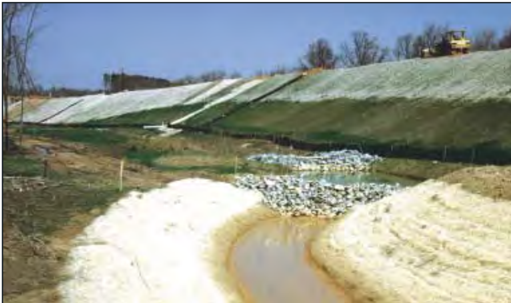
Figure 4.4 Phasing of rehabilitation is clearly evident on this batter
