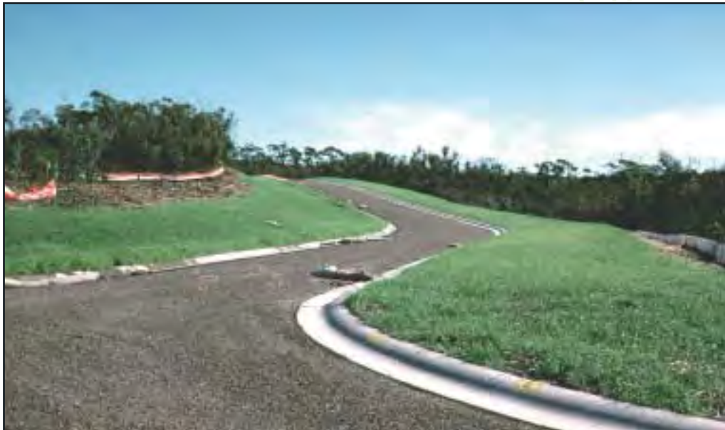
Figure 4.5 Recently rehabilitated lands at an urban subdivision near Sydney. Note the barrier mesh and sediment fencing still in position.
