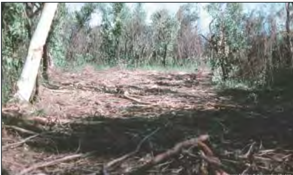
Figure 7.5 Effective mulching of a service easement using local brush
