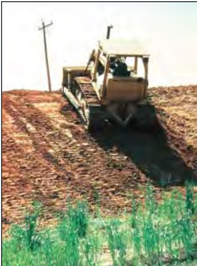
Figure 4.3(a) A track-walked slope (see footnote 4)
