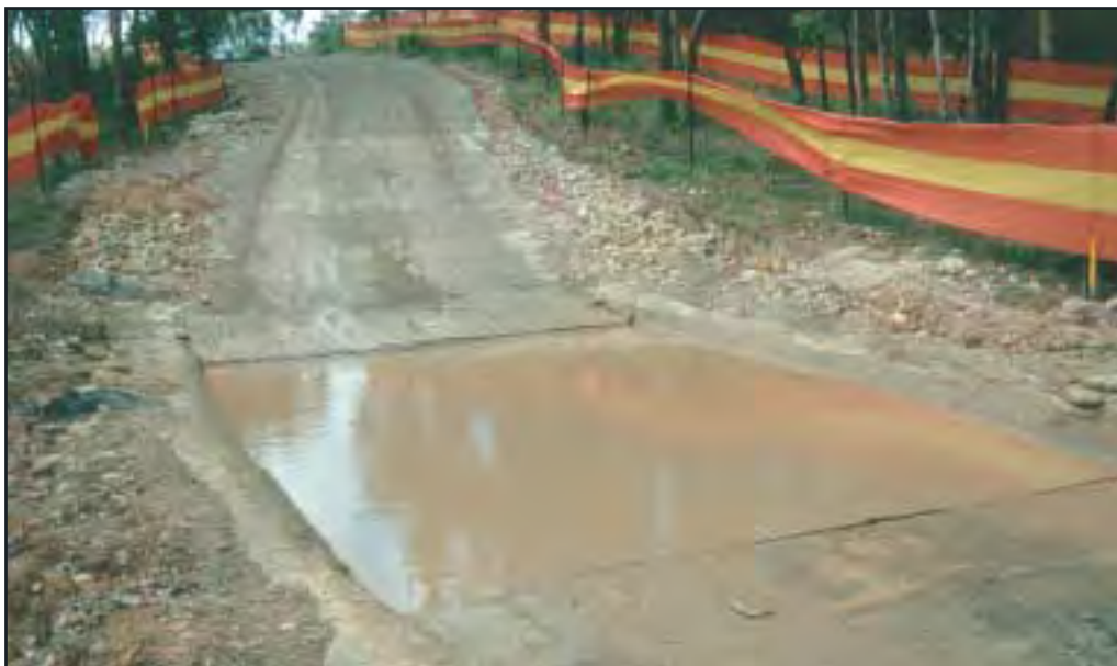
Figure 6.13 A simple wash-down system.
