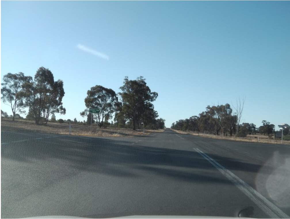
Photograph A.9 Wamboyne Road northbound, approaching Wamboyne Road/Girral Road/Blow Clear Road intersection
