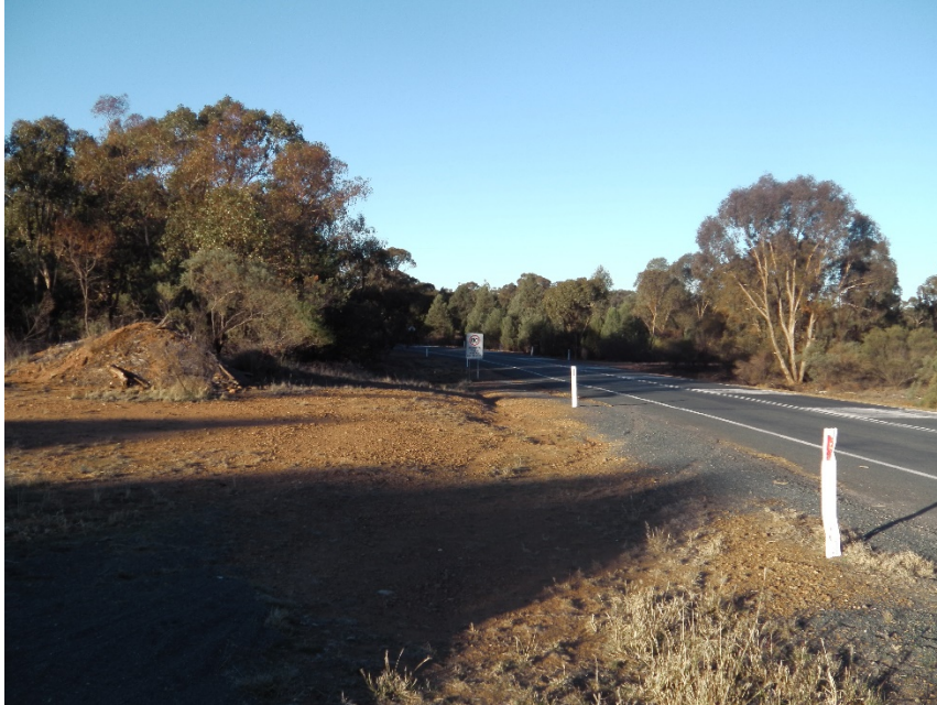
Photograph A.56 West Wyalong Condoblin Road/Ungarie Road/Wamboyne Road intersection – looking east towards Wamboyne Road
