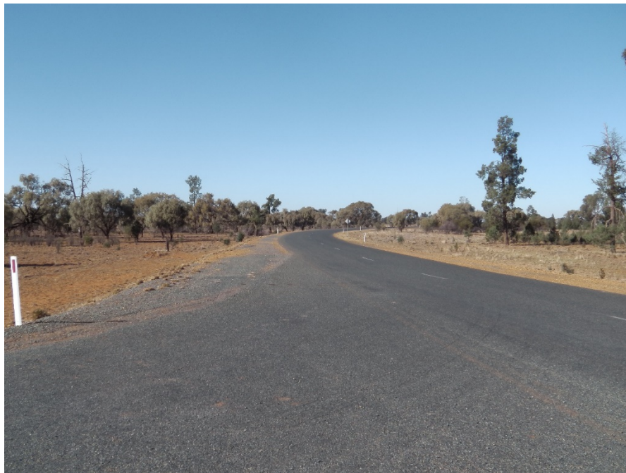
Photograph A.18 The Gipps Way, looking south from the The Gipps Way/Burcher Road intersection
