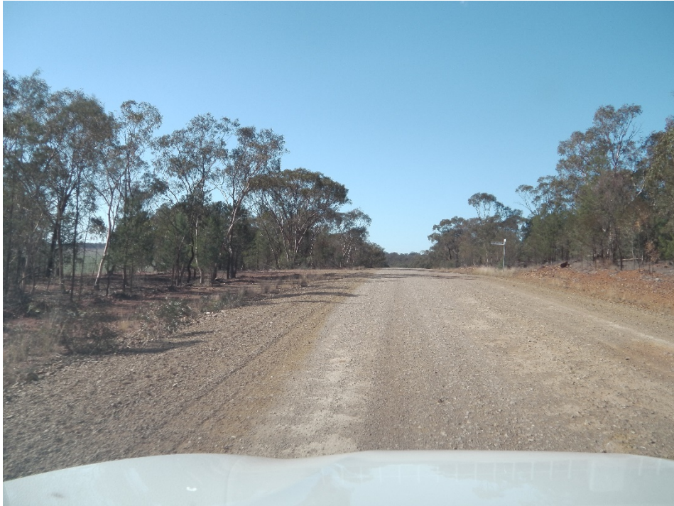
Photograph A.23 Lake Cowal Road eastbound, gravel road surface with good sight distance
