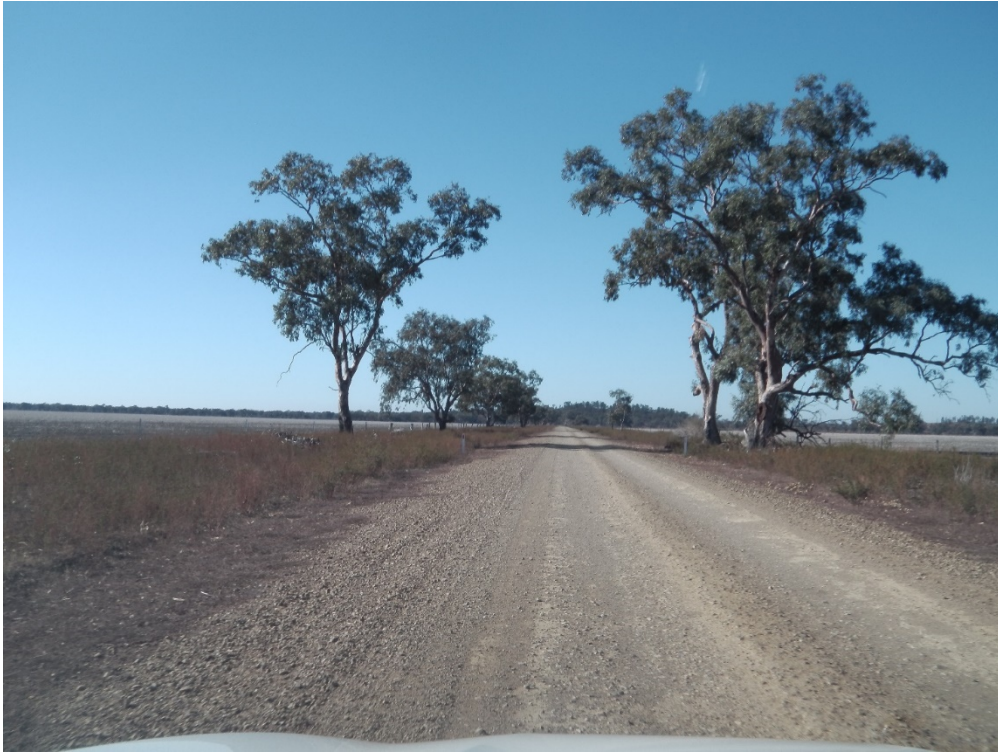
Photograph A.41 Bogies Island Road westbound, gravel surface in a relative open area
