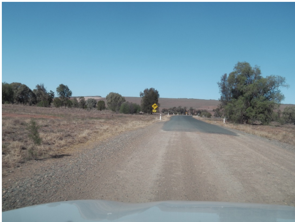
Photograph A.26 Lake Cowal Road southbound, approaching the section of sealed road surface
