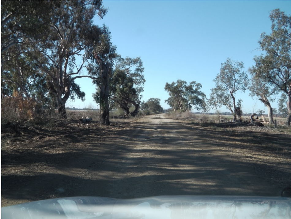
Photograph A.39 Bogies Island Road westbound, gravel surface
