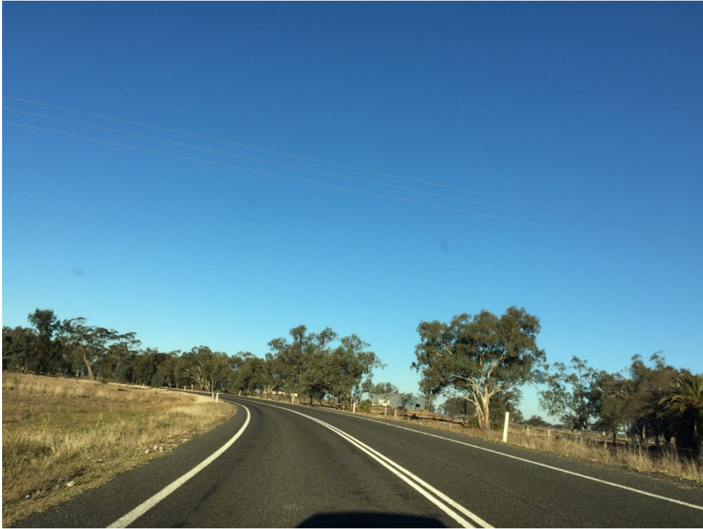
Photograph A.54 Lachlan Valley Way, approaching a road curve
