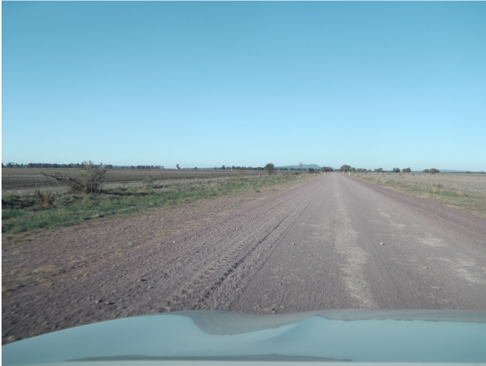
Photograph A.35 West Plains Road eastbound, unsealed section, long and straight
