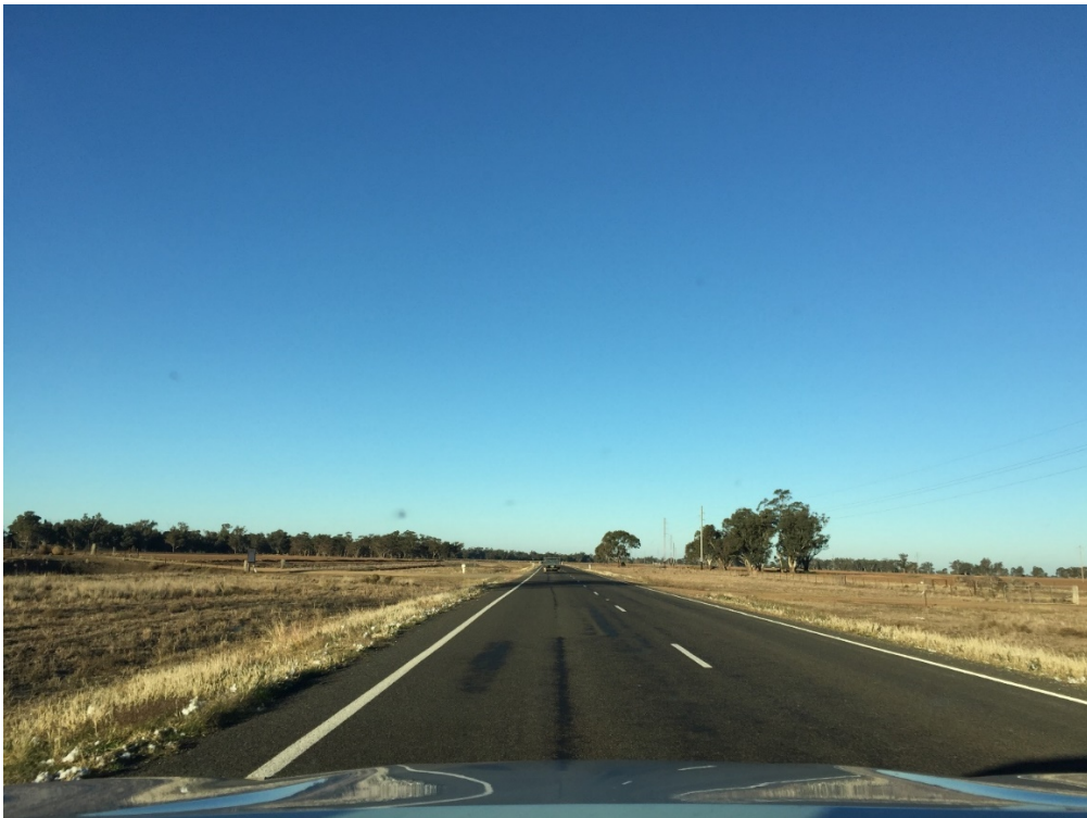
Photograph A.55 Lachlan Valley Way, long and straight road with excellent sight distance
