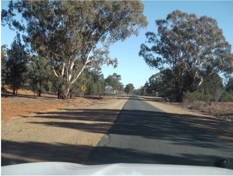
Photograph A.19 Burcher Road westbound, approaching the Burcher township
