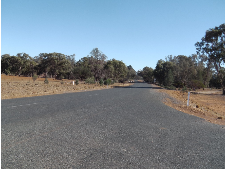
Photograph A.17 The Gipps Way, looking north from the The Gipps Way/Burcher Road intersection
