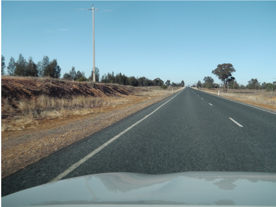
Photograph A.14 Bonehams Lane southbound, long straight road with excellent sight distance
