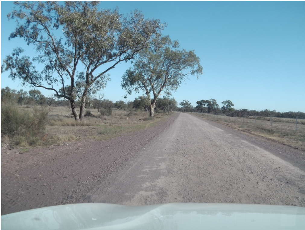
Photograph A.44 Lake Cowal Road westbound, gravel surface with excellent sight distance
