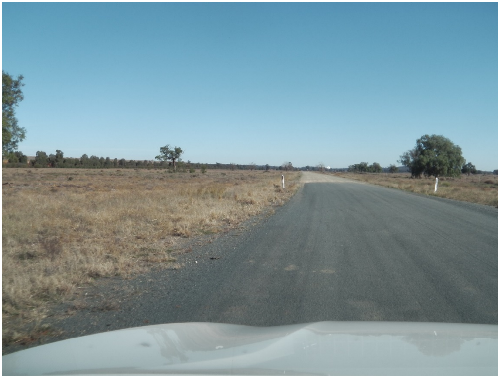
Photograph A.28 Lake Cowal Road southbound, road condition change from sealed to unsealed
