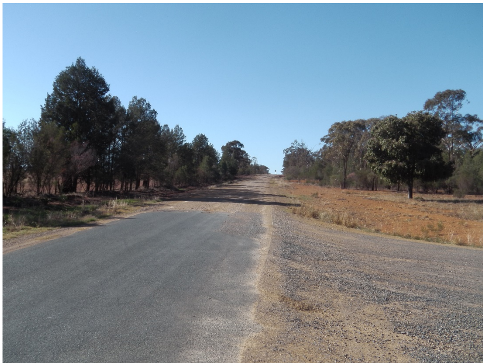
Photograph A.22 Bena Street eastbound, road condition change from sealed to unsealed surface
