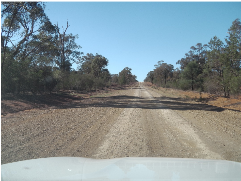
Photograph A.24 Lake Cowal Road eastbound, gravel road surface with excellent sight distance
