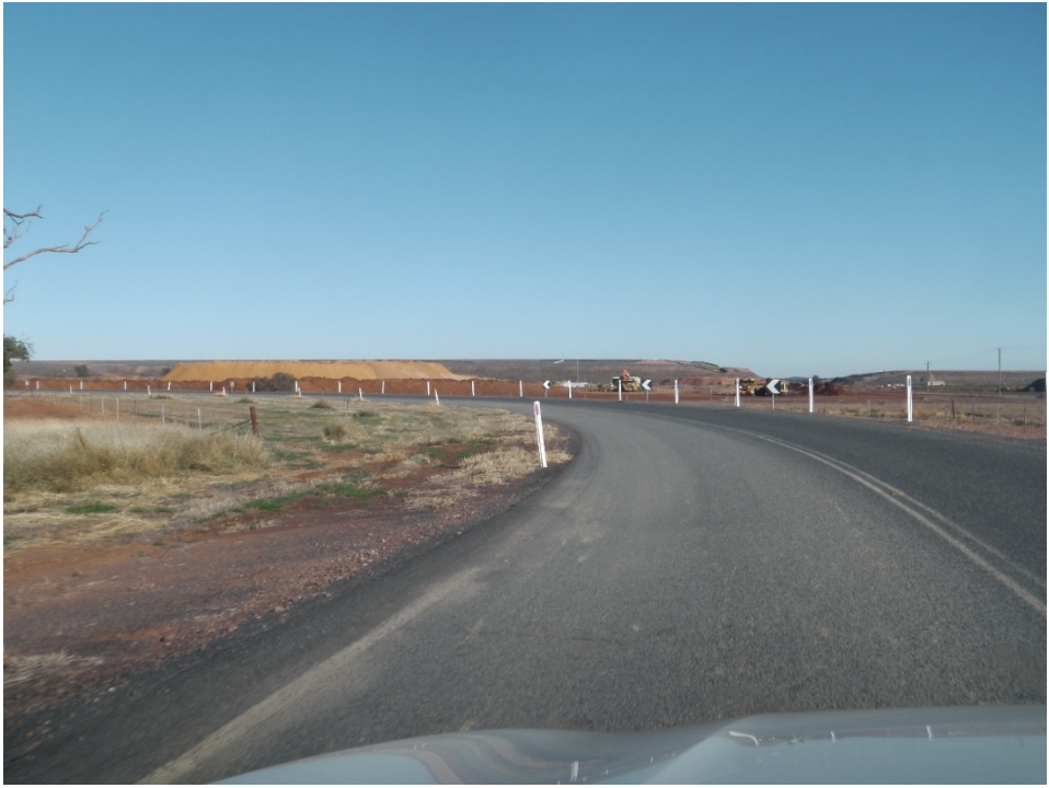
Photograph A.47 Mine access road, approaching a road curve
