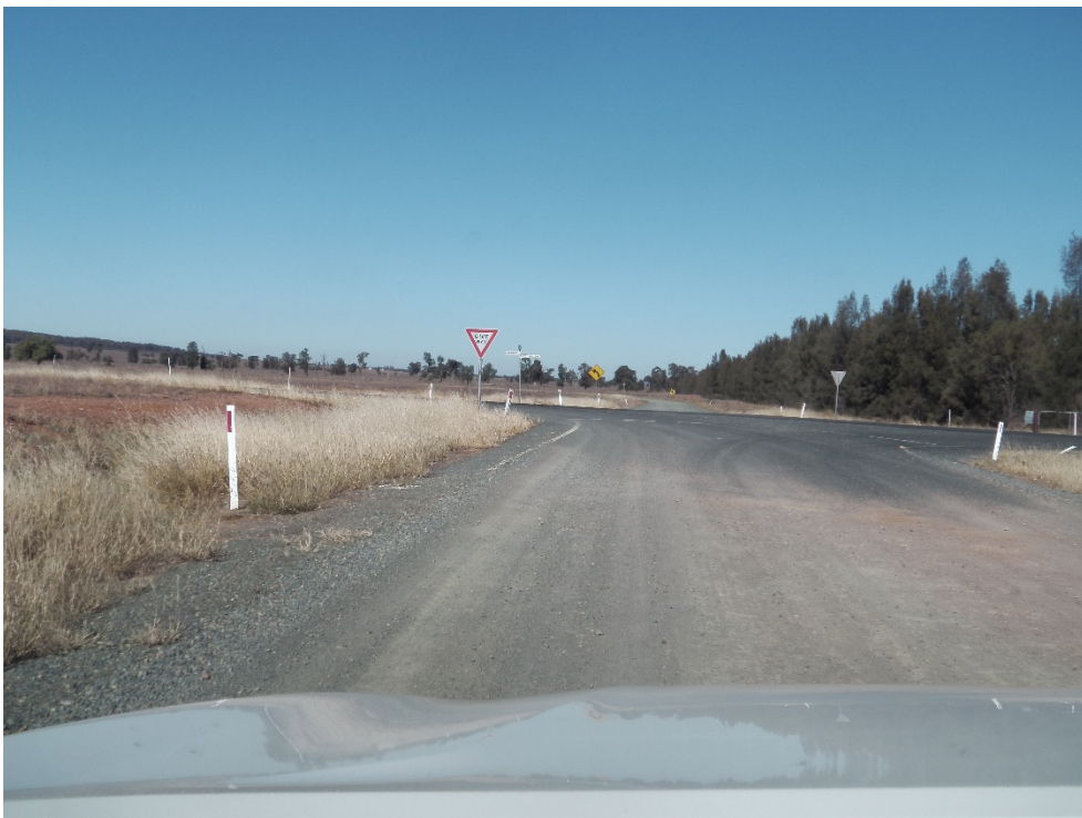
Photograph A.64 Looking south on Lake Cowal Road, approaching Bonehams Lane
