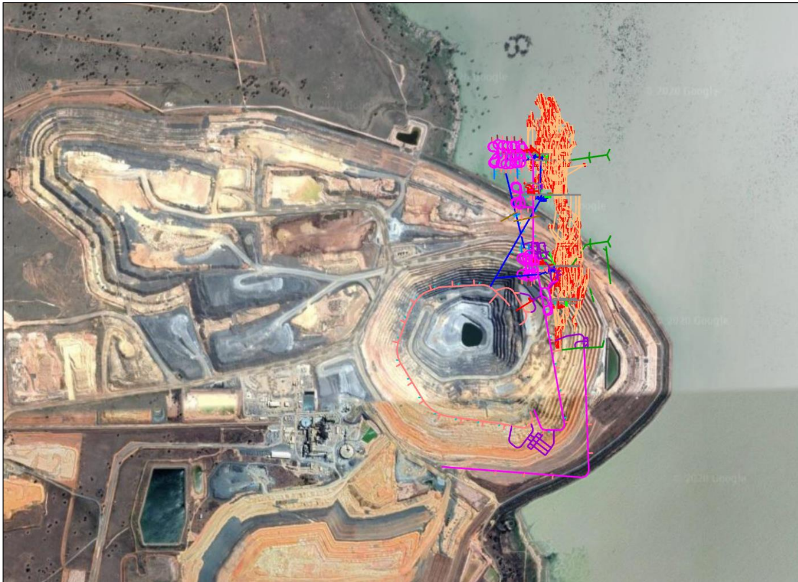
Figure 3-3: Aerial photo of the pit and Lake Cowal, with respect to the planned underground mine footprint
