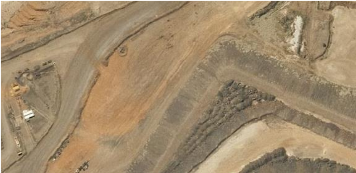
Map 7: Contractor demountable toilet block- irrigation area
