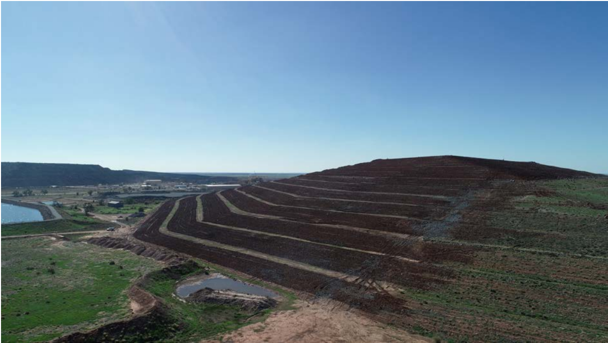
Plate 6: West End of Southern Waste Rock Emplacement (May 2019)
