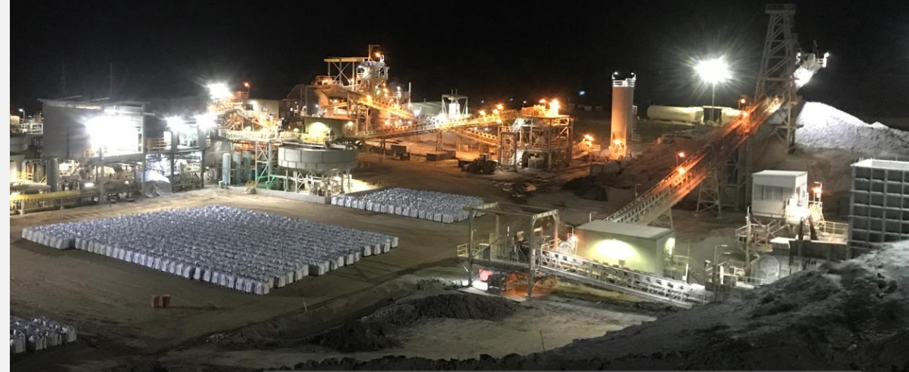
Mt Carlton processing plant
