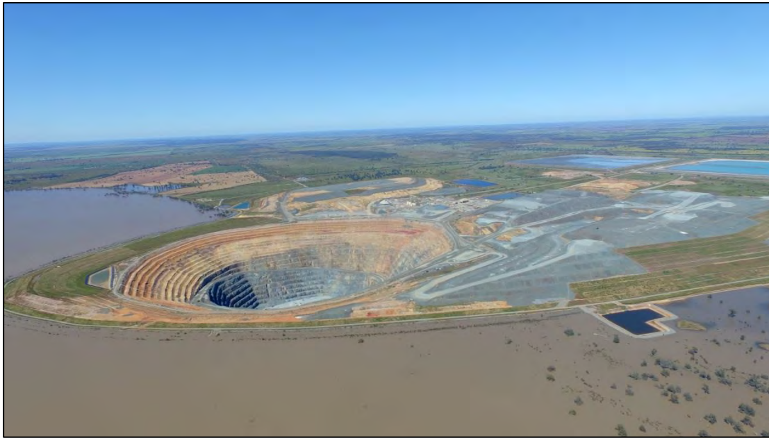
Plate 2: Aerial Photograph of the Lake Protection Bund
