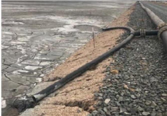
Droppers near the discharge point on eastern wall, Stage 5
