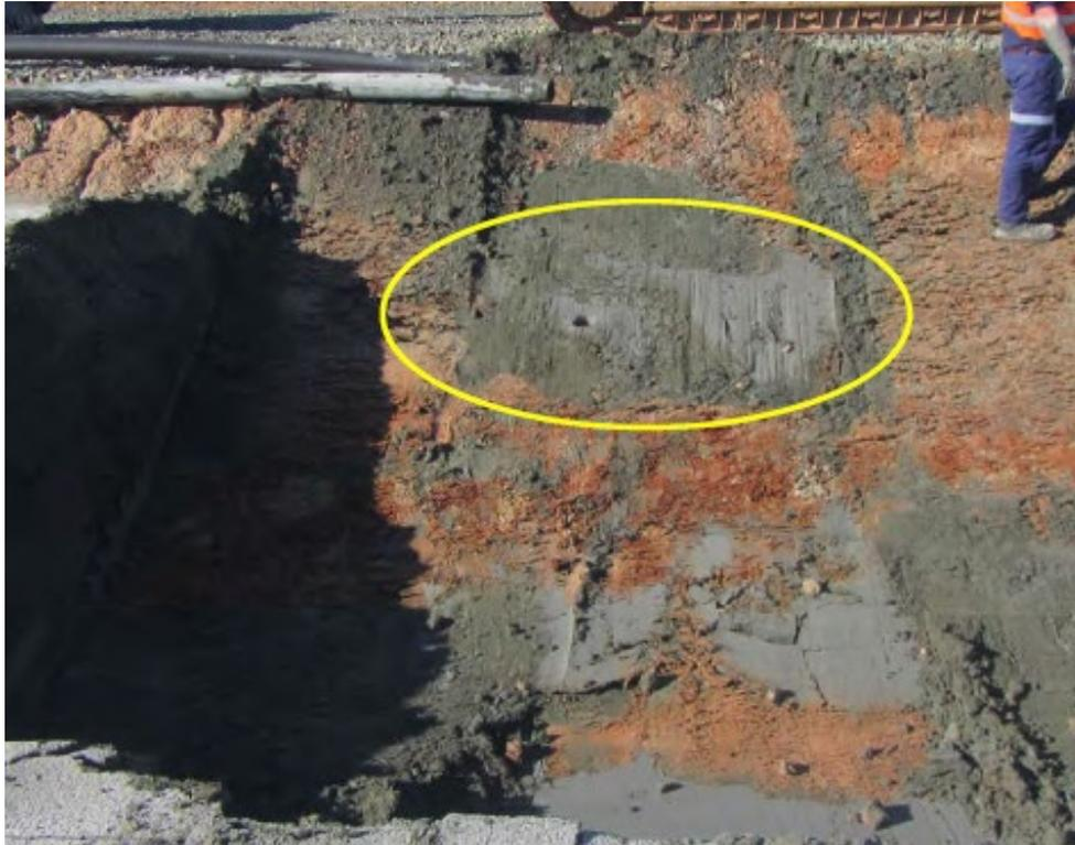
Clay liner with wet tailings exposed on eastern wall, Stage 5
