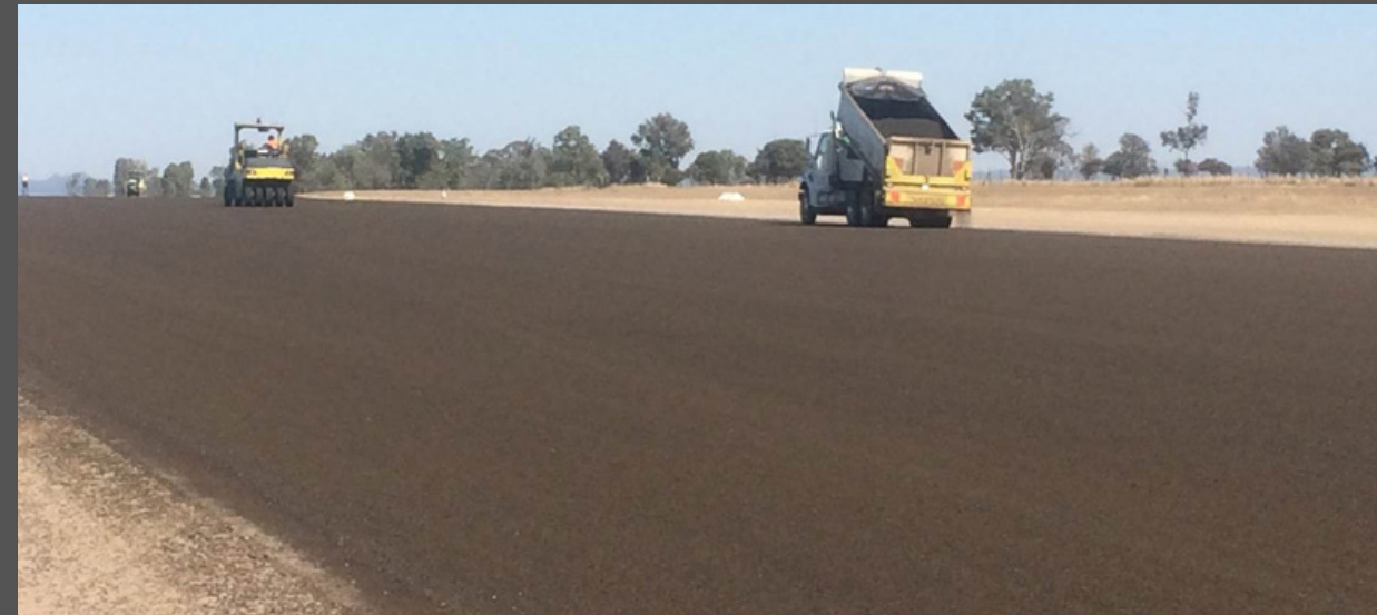
Construction of the aerodrome at Theodore
