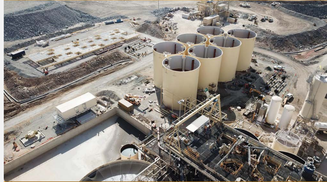
Float Tail Leach Project - Cowal
