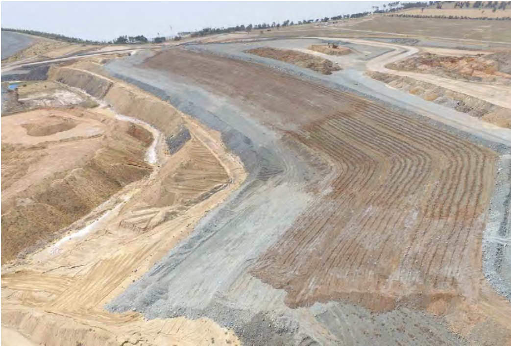
Plate 3: North Side of Southern Waste Rock Emplacement (November 2017)
