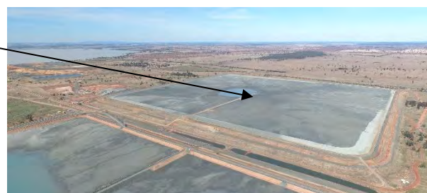
Southern Tailings Storage Facility (STSF) April 2017
