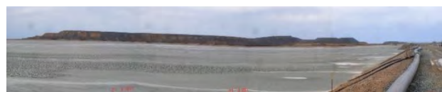
Northern Waste Rock Emplacement (NWRE) May 2016
