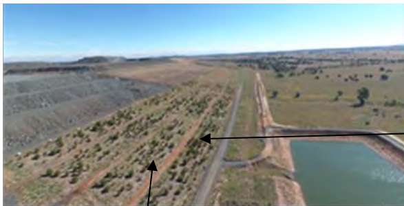
Aerial view of rehabilitated trials on the NWRE batter adjacent to Pond D1
