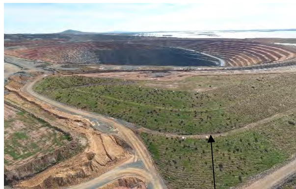
Perimeter Waste Emplacement rehabilitation on the outside lifts (above the Lake Protection Bund)
