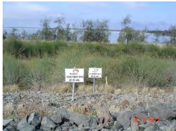
Temporary Isolation Bund - establishment of natural vegetation providing protection and stabilisation of the outer bund wall from the waters of Lake Cowal (when the lake bed was inundated).
