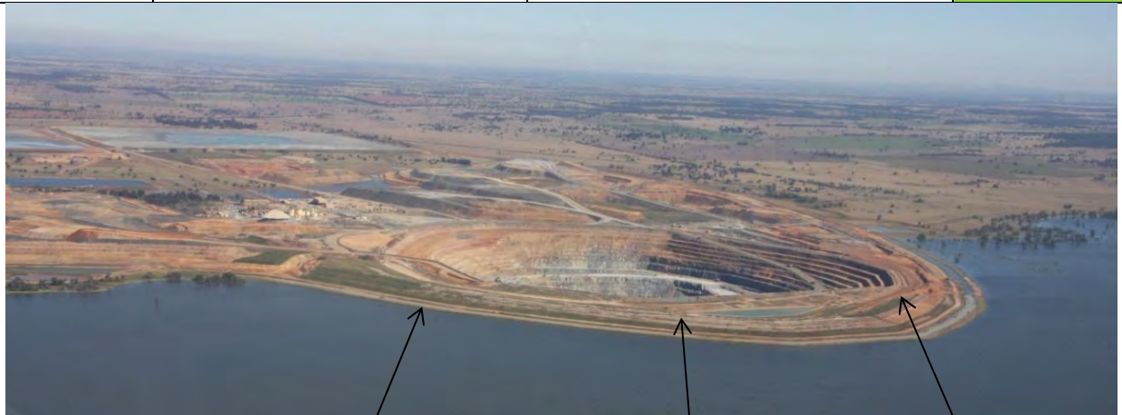
Cowal Gold Mine pit showing temporary isolation bund, lake protection bund and perimeter waste emplacement (2016).
