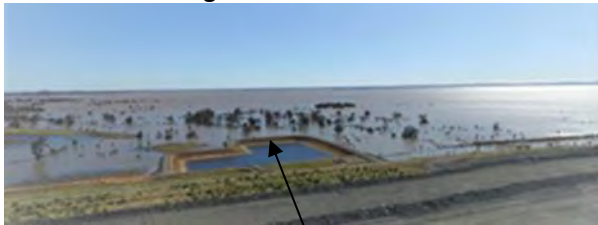
Bund wall protection of Pond D1 during the peak water level of Lake Cowal in 2016.
