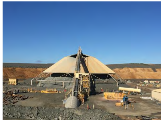
Plate 4-1: Cover Over the Coarse Ore Stockpile
