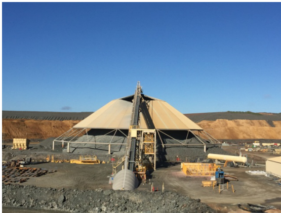
Plate 4-1: Cover Over the Coarse Ore Stockpile
