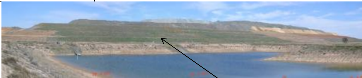
Perimeter Waste Emplacement rehabilitation trials of the outside lifts (above the Lake Protection Bund)
