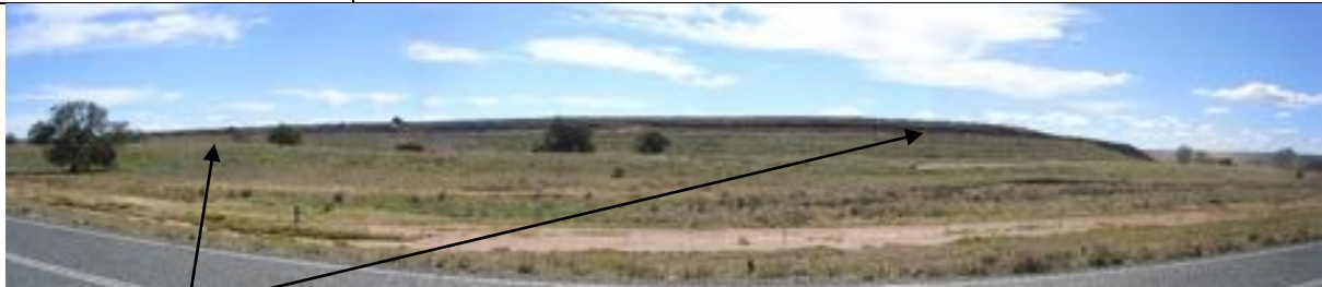
STSF outer batter being strengthened with rock butress to meet the Tailings Management Standard for earthquake stability.
