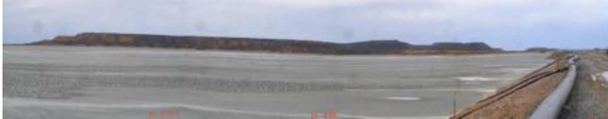
NTSF receiving tailings from mid-2014 to April 2015.
