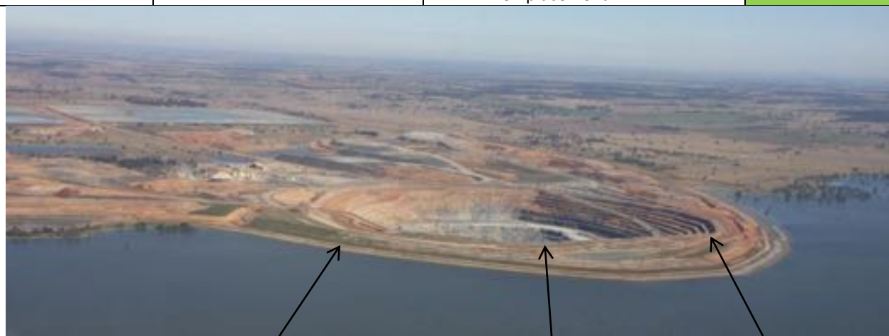
Cowal Gold Mine pit showing temporary isolation bund, lake protection bund and perimeter waste emplacement.
