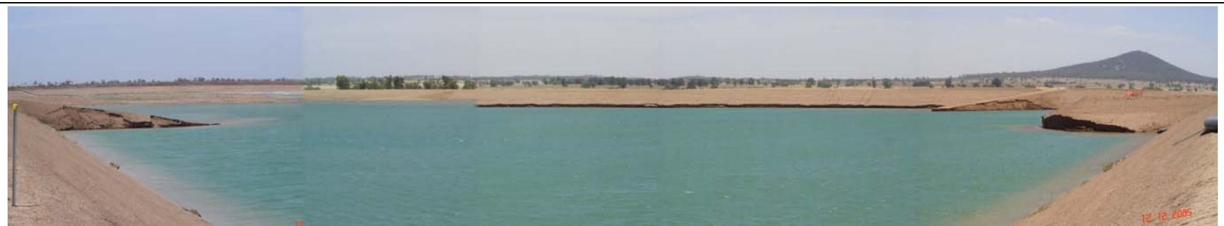
Plate K: Northern Tailings Storage Facility containing water pumped from the mine pit dewatering bores and groundwater from the Bland palaeochannel borefield.
