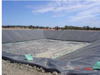
Plate 2: Contained Water Storage D6 – HDPE lined.
