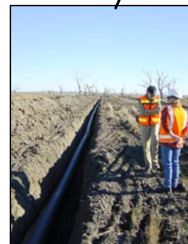
Plate 6: Pipeline trench across Lake Cowal.
