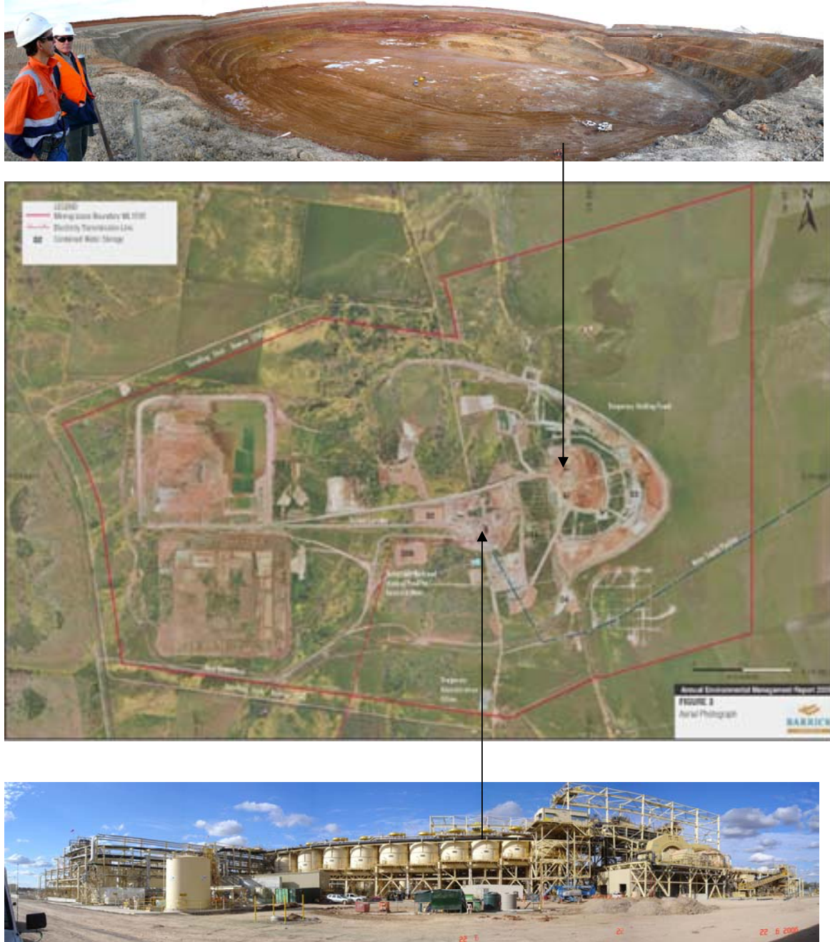
Plate 8: Process plant 22 June 2006 during commissioning period.
