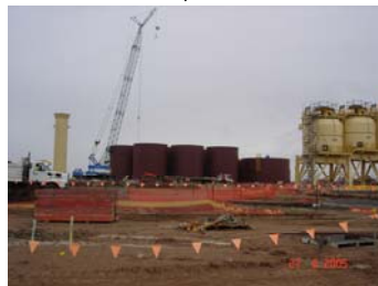
Plate 5: Bulk storage tanks installation adjacent to process plant
