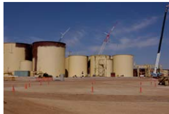
Plate 5: Bulk storage tanks installation adjacent to process plant
