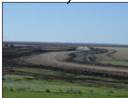
Plate 5: Commencement of Temporary Isolation Bund.
