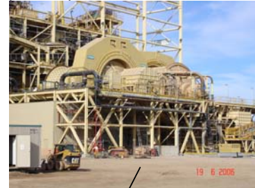
Plate 3: Ball Mill fabrication for the process plant – Dec 2005
