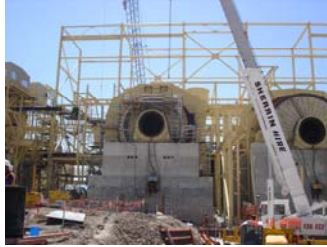
Plate 2: Ball Mill fabrication for the process plant – December 2005
