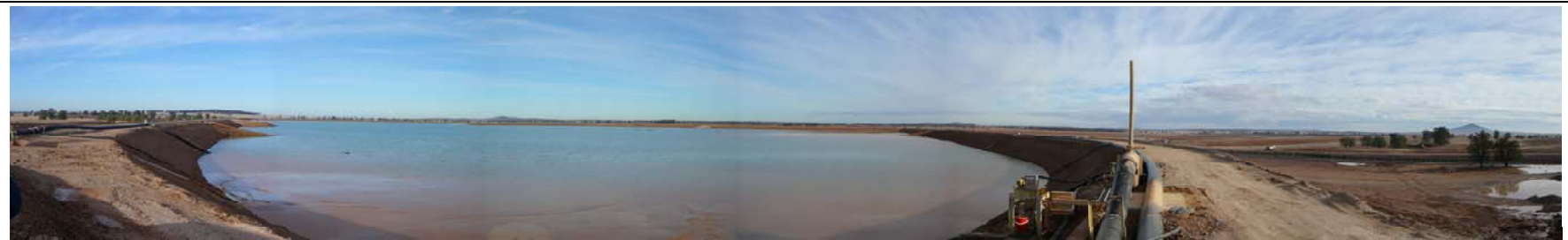
Plate J: Southern Tailings Storage Facility 23 June 2006, receiving tailings from the process plant commissioning, and decant water is returned to the process plant for reuse.
