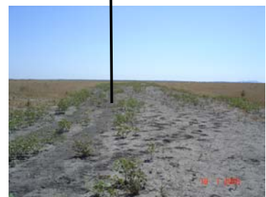
Plate 6: Rehabilitated pipeline trench across Lake Cowal January 2005.
