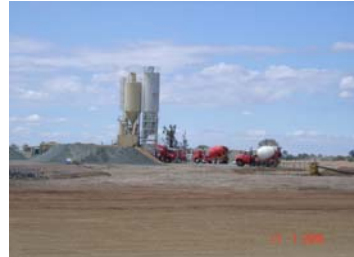
Plate 3: Concrete Batch Plant near Process Plant Area
