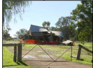
Plate 3: Heritage building with protective fencing
