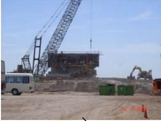
Plate 1: Crusher in excavation – December 2005
