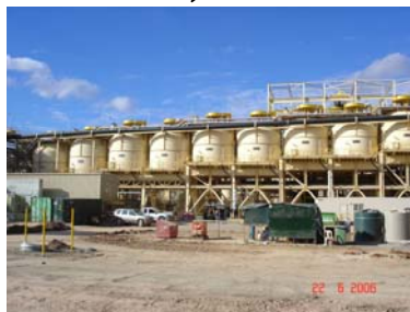
Plate 4: Flotation tanks – process plant - June 2006
