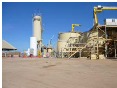
Plate 5: Bulk storage tank installation process plant – June 2006
