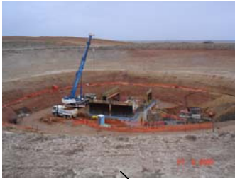
Plate 1: Crusher in excavation – June 2005
