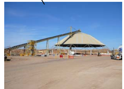
Plate 6: Covered ore stockpile area adjacent to the process plant
