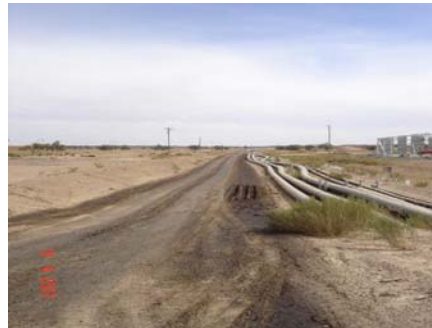
PetroTac coating of roads within the mine lease – 18 April 2007
