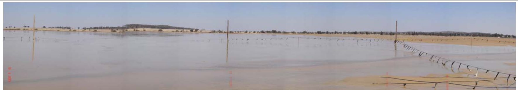
Southern Tailings Storage Facility 18 April 2007 with tailings from the first 12 months of operation of the CGP processing plant, with decant water returned to the plant for reuse.
