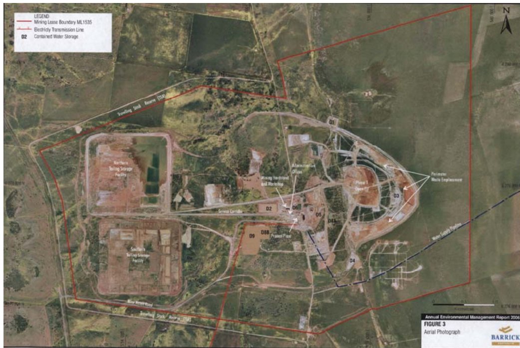
Plate 1: Cowal Gold Project Mining Lease Layout – Aerial Photograph 2006
