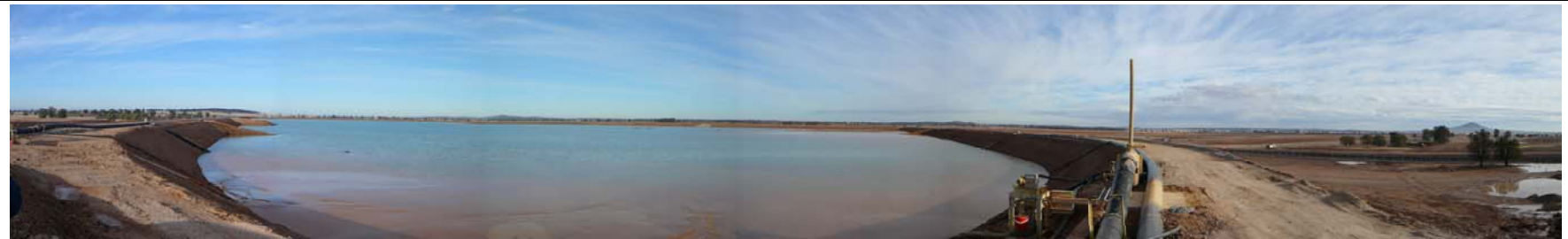
Southern Tailings Storage Facility 23 June 2006, receiving tailings from the process plant commissioning. Decant water is returned to the process plant for reuse.
