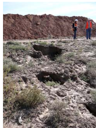
Plate 3: Erosion from reactive soils on the access track on the southern side of the Lake Protection bund.
