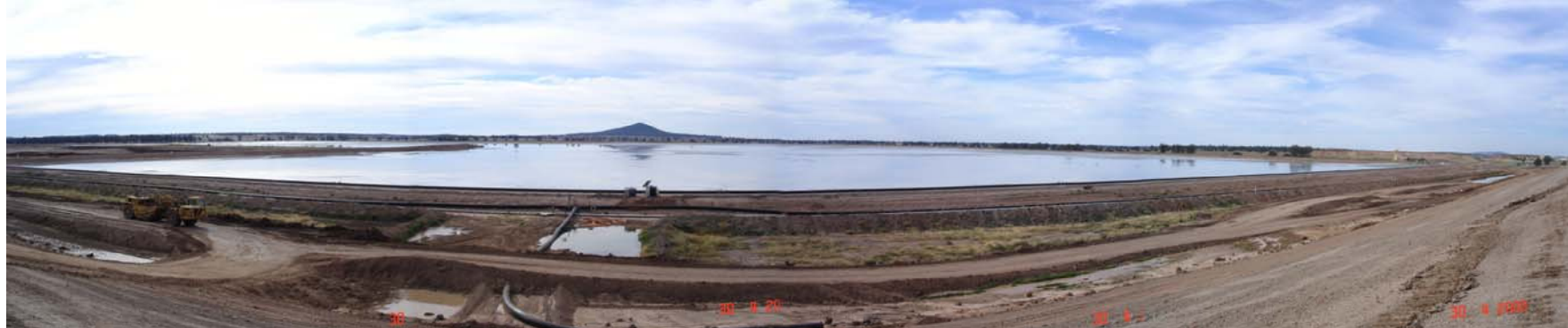
Northern Tailings Storage Facility (looking north from the 3m lift of the STSF) May 2008
