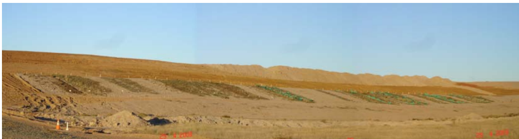
Plate 5: Rehabilitation trials on the mine pit batters using native seed stock/tube stock
