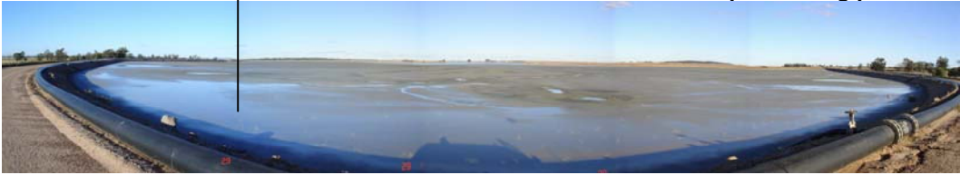
Northern Tailings Emplacement Area (from north western corner) May 2008
