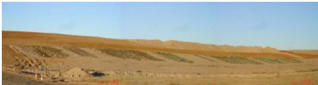
Plate 5: Rehabilitation trials on the mine pit batters using mulch, subsoil, rock and native seed stock/tube stock
