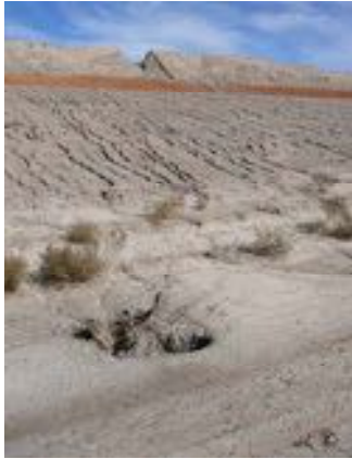
Plate 2: Erosion on the lake protection bund from rainfall runoff.
