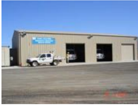
CGP Emergency Response Centre
