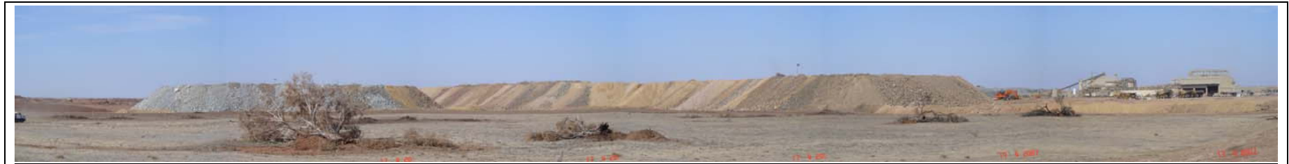
Northern waste rock emplacement area– April 2007
