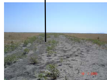
Plate 6: Rehabilitated pipeline trench across Lake Cowal January 2005.
