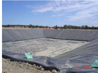
Plate 2: Contained Water Storage D6 – HDPE lined.
