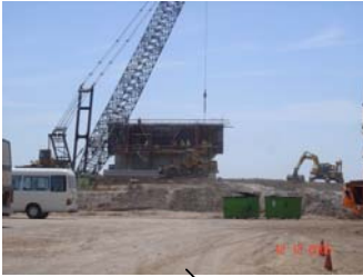
Plate 1: Crusher in excavation – December 2005
