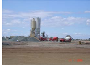
Plate 3: Concrete Batch Plant near Process Plant Area
