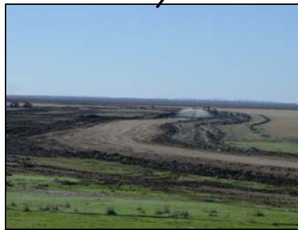
Plate 5: Commencement of Temporary Isolation Bund.
