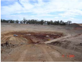
Plate 1: Crusher pit excavation – January 2005
