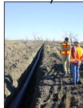
Plate 6: Pipeline trench across Lake Cowal.
