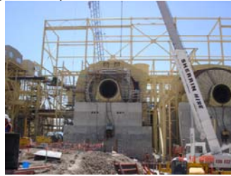
Plate 2: Ball Mill fabrication for the process plant – December 2005
