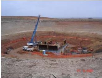
Plate 1: Crusher in excavation – June 2005
