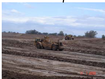
Plate 4: Northern Tailings Storage Facility establishment January 2005.
