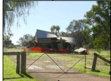
Plate 3: Heritage building with protective fencing
