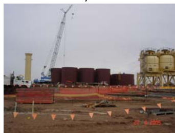
Plate 5: Bulk storage tanks installation adjacent to process plant
