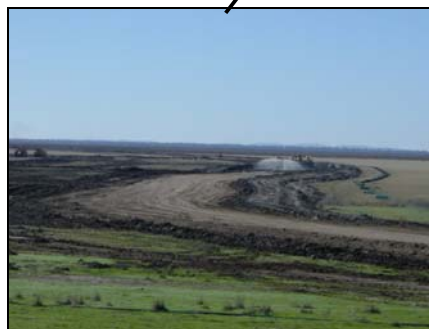
Plate 5: Commencement of Temporary Isolation Bund.
