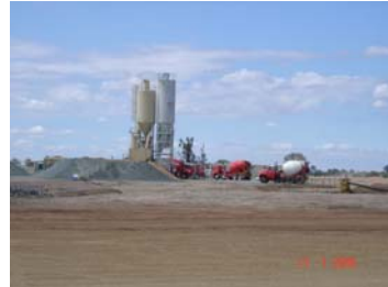
Plate 3: Concrete Batch Plant near Process Plant Area
