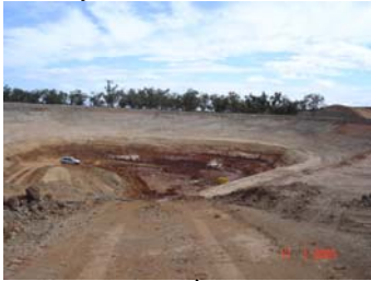
Plate 1: Crusher pit excavation – January 2005
