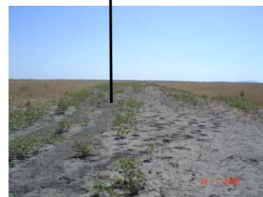
Plate 6: Rehabilitated pipeline trench across Lake Cowal January 2005.
