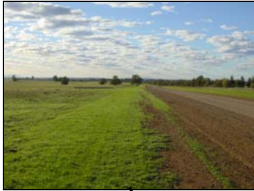
Plate 1: TSR and new road June 2004.
