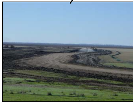
Plate 5: Commencement of Temporary Isolation Bund.
