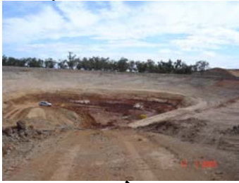
Plate 1: Crusher pit excavation – January 2005
