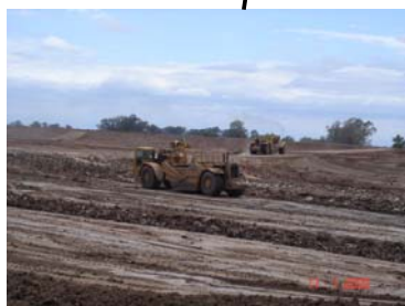
Plate 4: Northern Tailings Storage Facility establishment January 2005.
