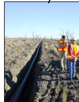
Plate 6: Pipeline trench across Lake Cowal.
