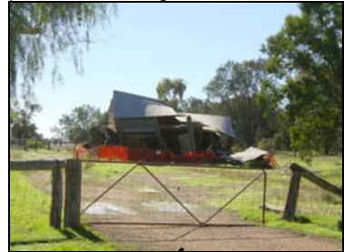
Plate 3: Heritage building with protective fencing
