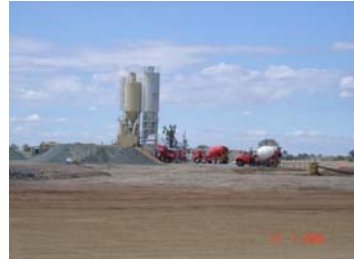
Plate 3: Concrete Batch Plant near Process Plant Area
