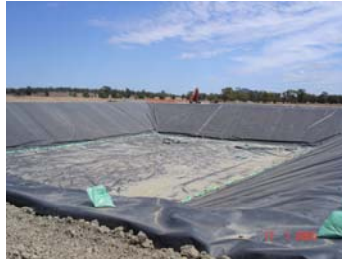
Plate 2: Contained Water Storage D6 – HDPE lined.
