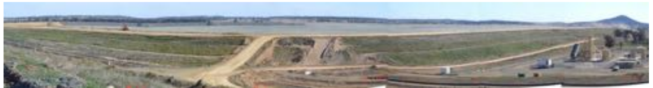
NTSF construction of the new lift (May 2014)
