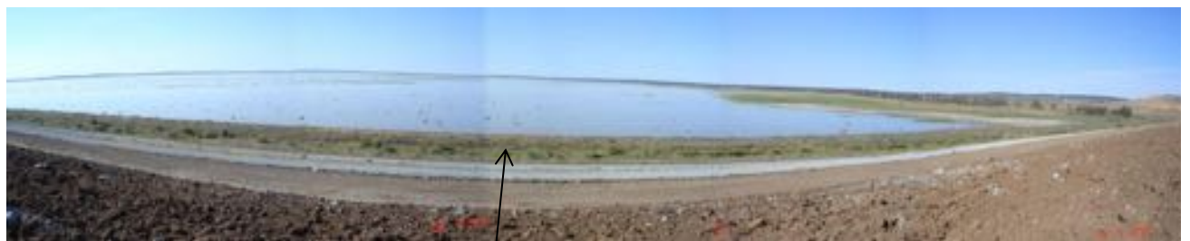
Temporary Isolation Bund establishment of natural vegetation providing protection of the outer bund wall from wind / wave erosion resulting from the waters of Lake Cowal.
