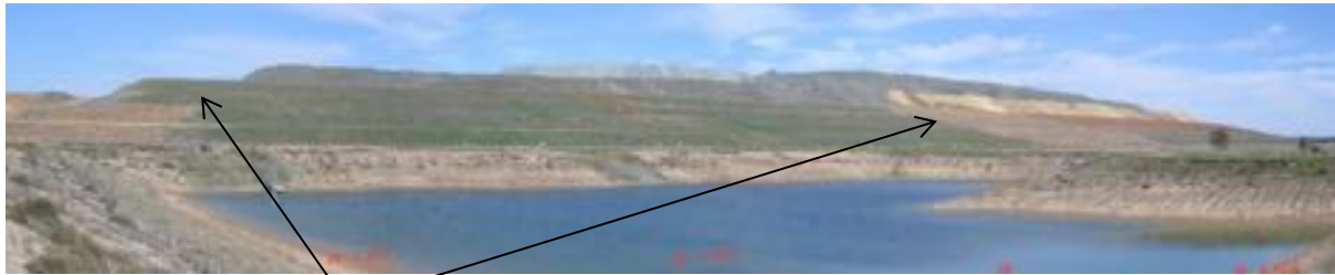
Plate 10: Rehabilitation trial on lake side overburden emplacement with contouring and using straw bale substrate to control erosion and retain soil for vegetation establishment
