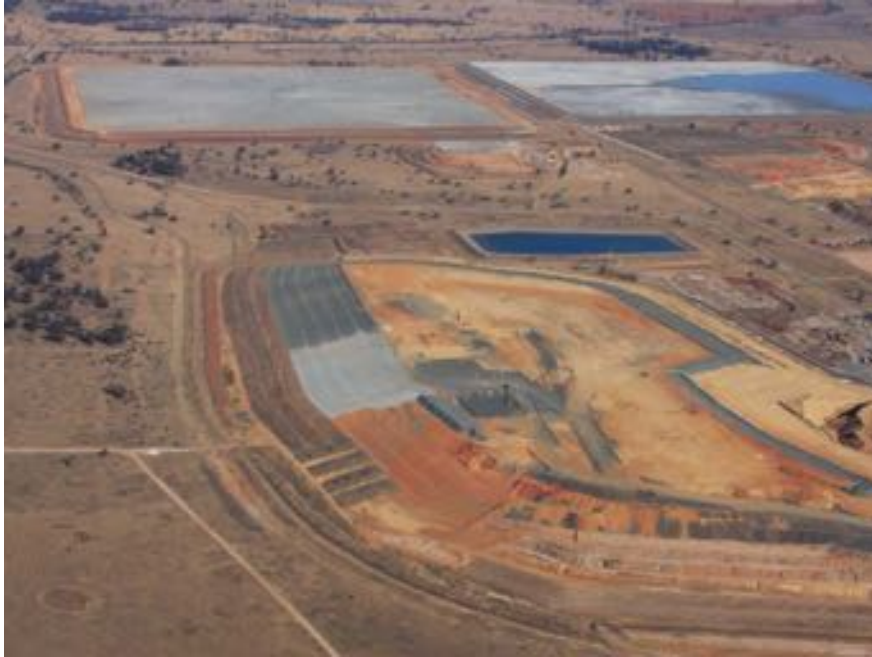
Plate 6: Rehabilitation works continuing on Southern Waste Rock Emplacement (March 2015).
