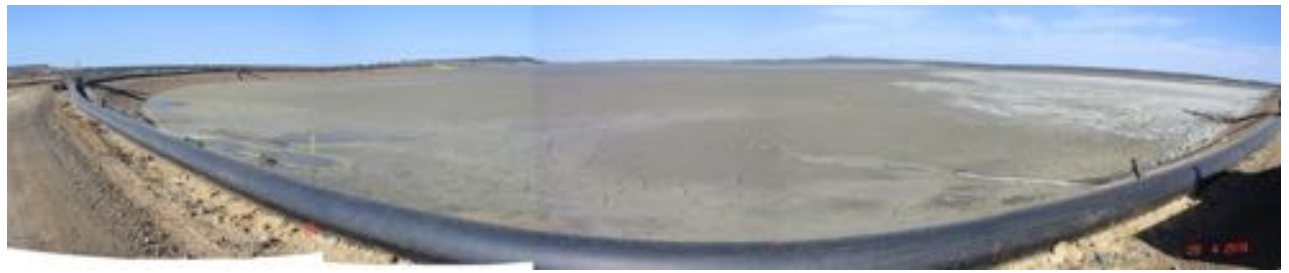
STSF in use May 2014 with recovery of tailings water for use in the process plant.
