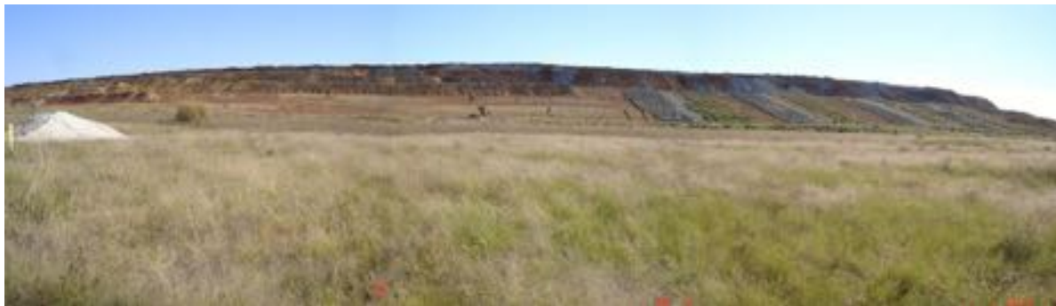
Plate 11: Rehabilitation trials along the southern wall of the Southern Waste Emplacement Area.
