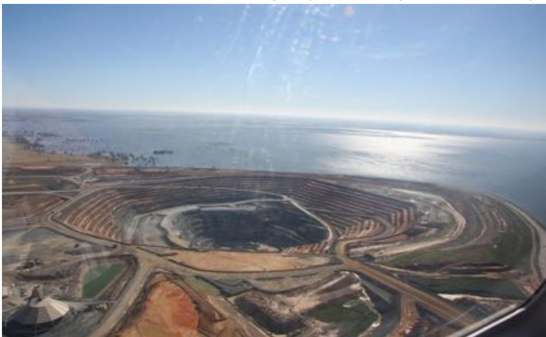
Plate 1: CGM with Lake Cowal waters beyond (Photo courtesy of Barrick Australia)
