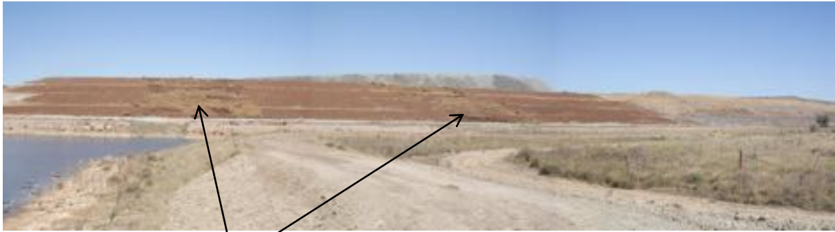
Plate 3: Rehabilitation trial on lake side overburden emplacement with contouring and using straw bale substrate to control erosion and retain soil for vegetation establishment
