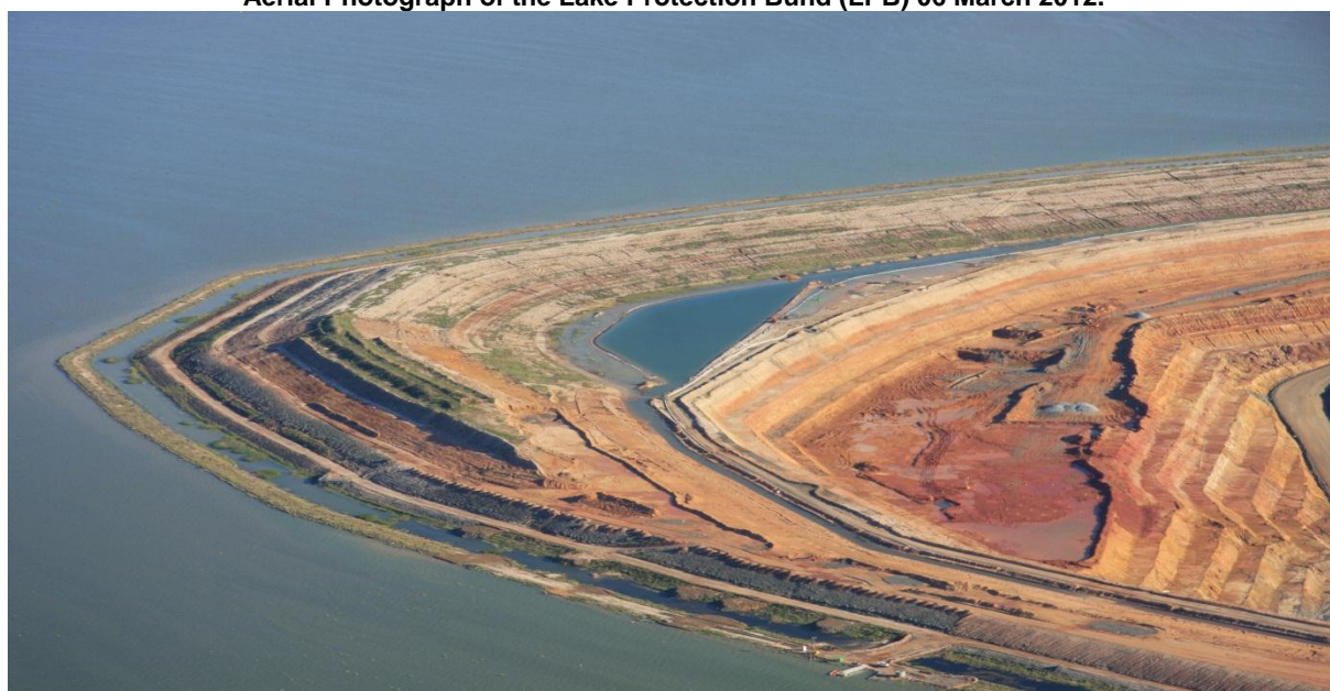
Plate 3 Aerial Photograph of the Lake Protection Bund (LPB) 06 March 2012.
