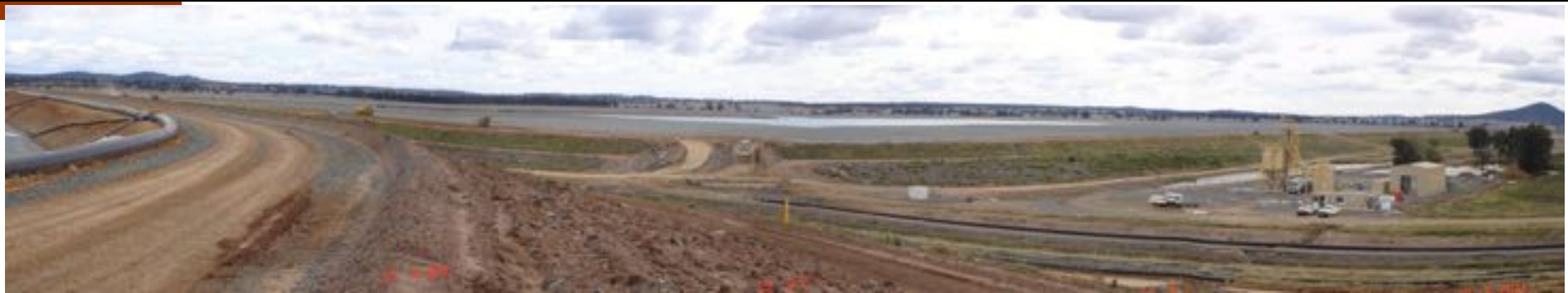
Plate 9: Northern Tailing Storage Facility (looking north from the north east corner of the STSF) April 2011
