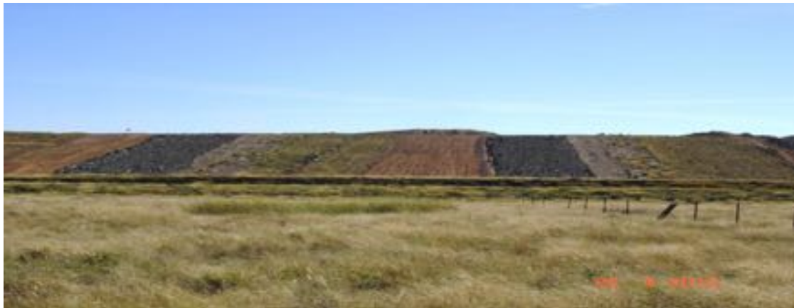
Plate 3: Rehabilitation trials along the southern wall of the Southern Waste Emplacement Area
