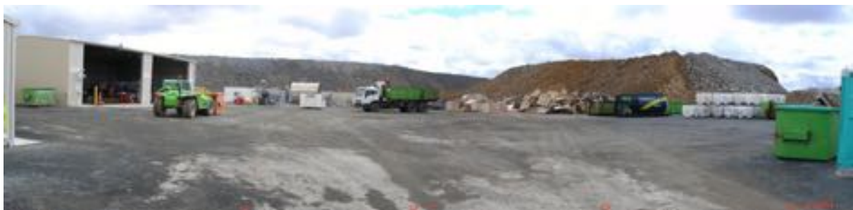
Plate 6: J R Richards waste management area with segregated wastes – CGP April 2011
