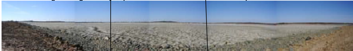
Southern Tailings Emplacement Area April 2010 – dry tailings preparation of top wall for new lift.
