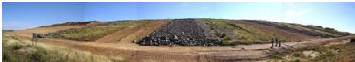
Rehabilitation trials using mulch, topsoil, subsoil, rock and native seed application
