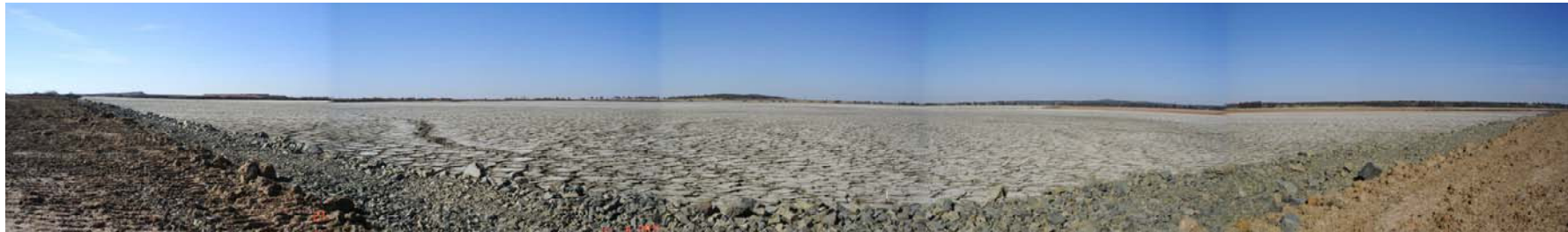
Southern Tailing Storage Facility – dried tailings ready for construction of the next lift (looking southeast April 2010).
