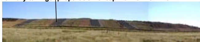
Southern Tailings Emplacement Area April 2010 – dry tailings preparation of top wall for new lift.
