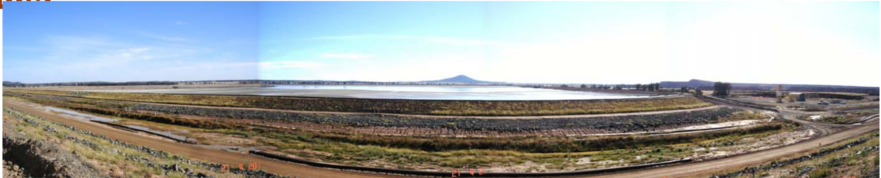
Northern Tailing Storage Facility (looking north from the north east corner of the STSF) April 2010
