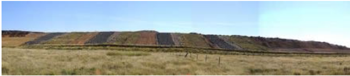
Rehabilitation trials along the southern wall of the Southern Waste Emplacement Area
