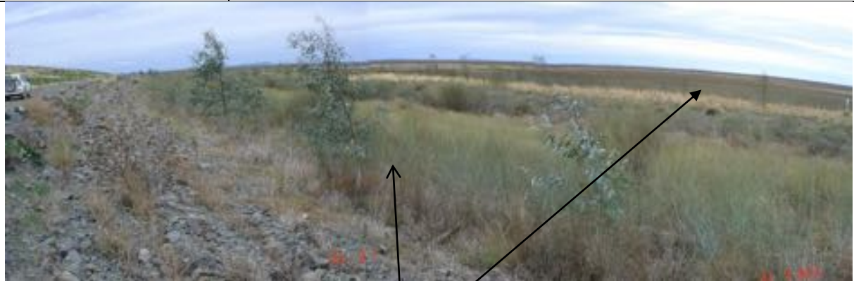
Temporary Isolation Bund - establishment of natural vegetation providing protection and stabilisation of the outer bund wall from the waters of Lake Cowal (when the lake bed was inundated).
